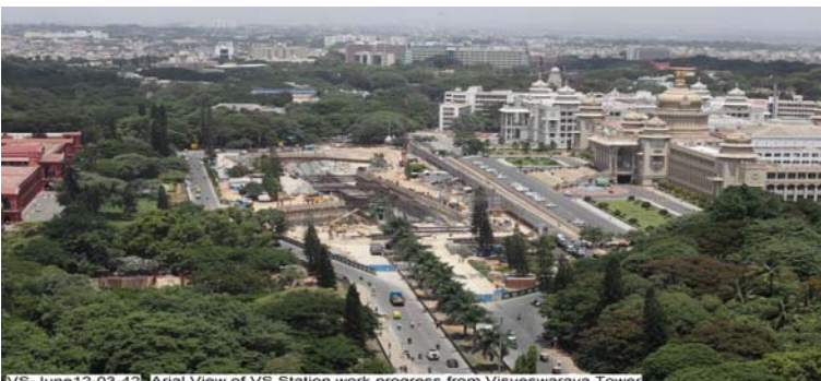
ARIAL VIEW OF THE VIDHANA Soudha STATION WORK PROGRESS
